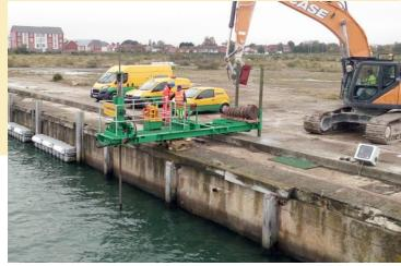
A hitch was fitted to the cantilever frame to allow an excavator to secure the frame and provide the reaction force during the push.
